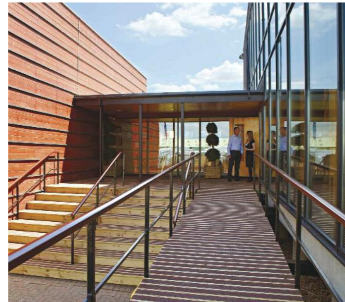
WALKWAYS AND STEPS, METSÄ WOOD, (BOSTON)
