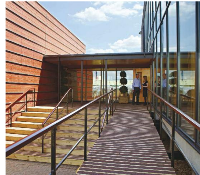
WALKWAYS AND STEPS, METSÄ WOOD, (BOSTON)
