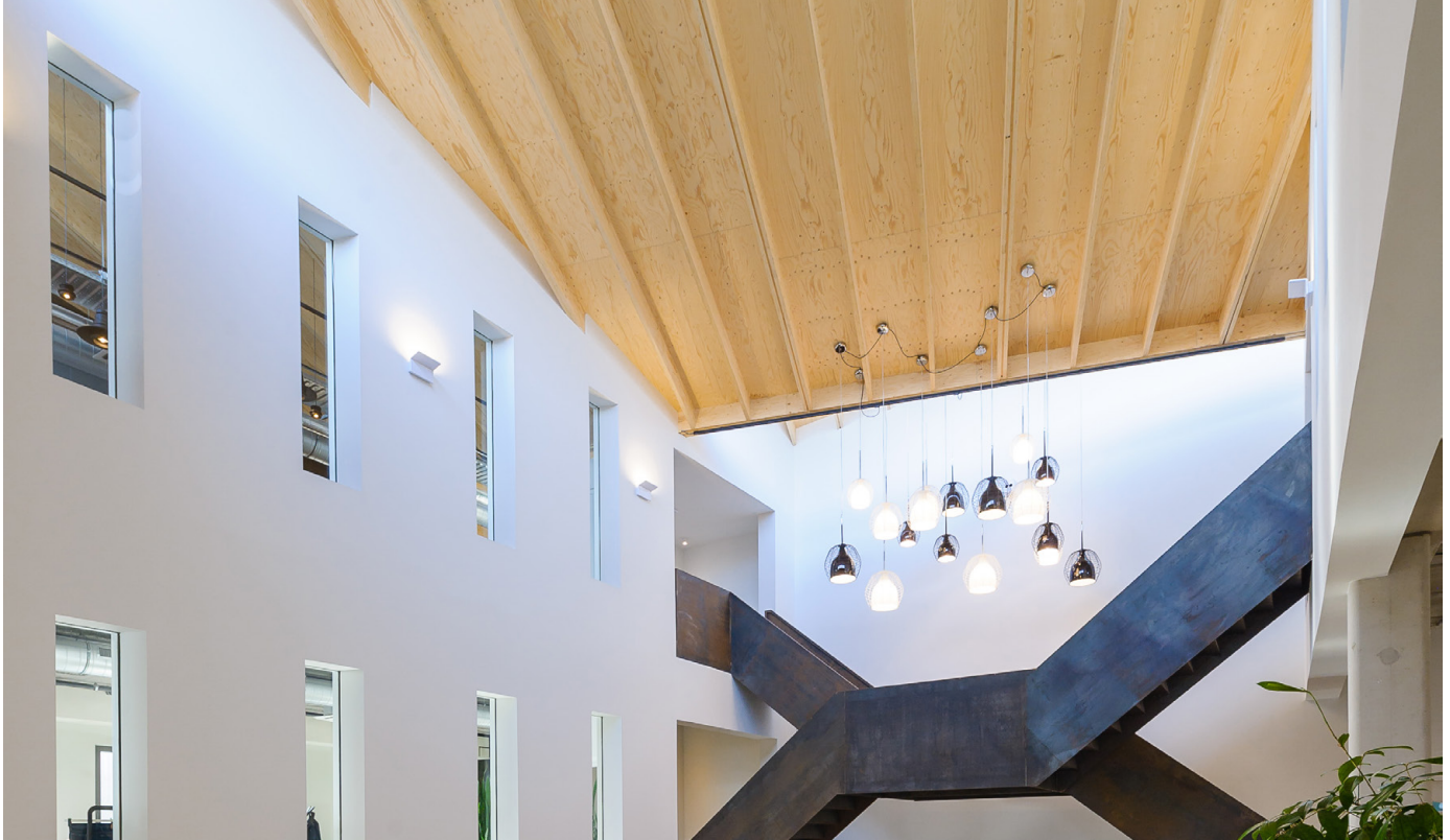
Kerto-Ripa® in roof structure
