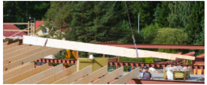
Figure 3. Kerto-S roof beam cut to special shape.
